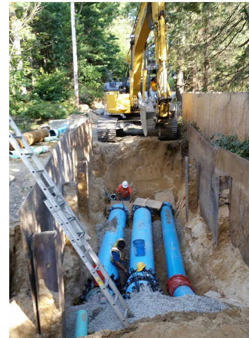
PVC Force Main Installation CASE STUDY NO.1
