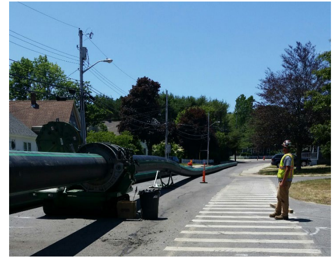
HDPE Force Main For Slip-Lining CASE STUDY NO.1
